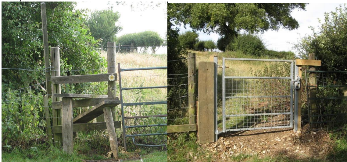
Footpath 25: before and after
