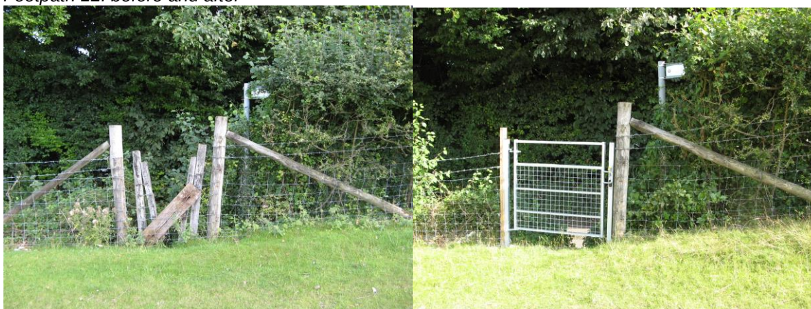
Footpath 12: before and after
